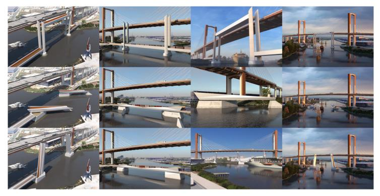
Draft of the Preliminary Design for a Movable Railway Bridge to Provide Access, Crossing the Port Basin, to the Container Terminal at the Port of Seville
